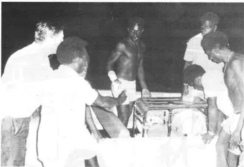
Plate 13: The generator being loaded on to a small boat.
