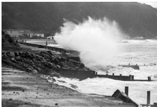
The new seawall being pounded by high seas, 1977
