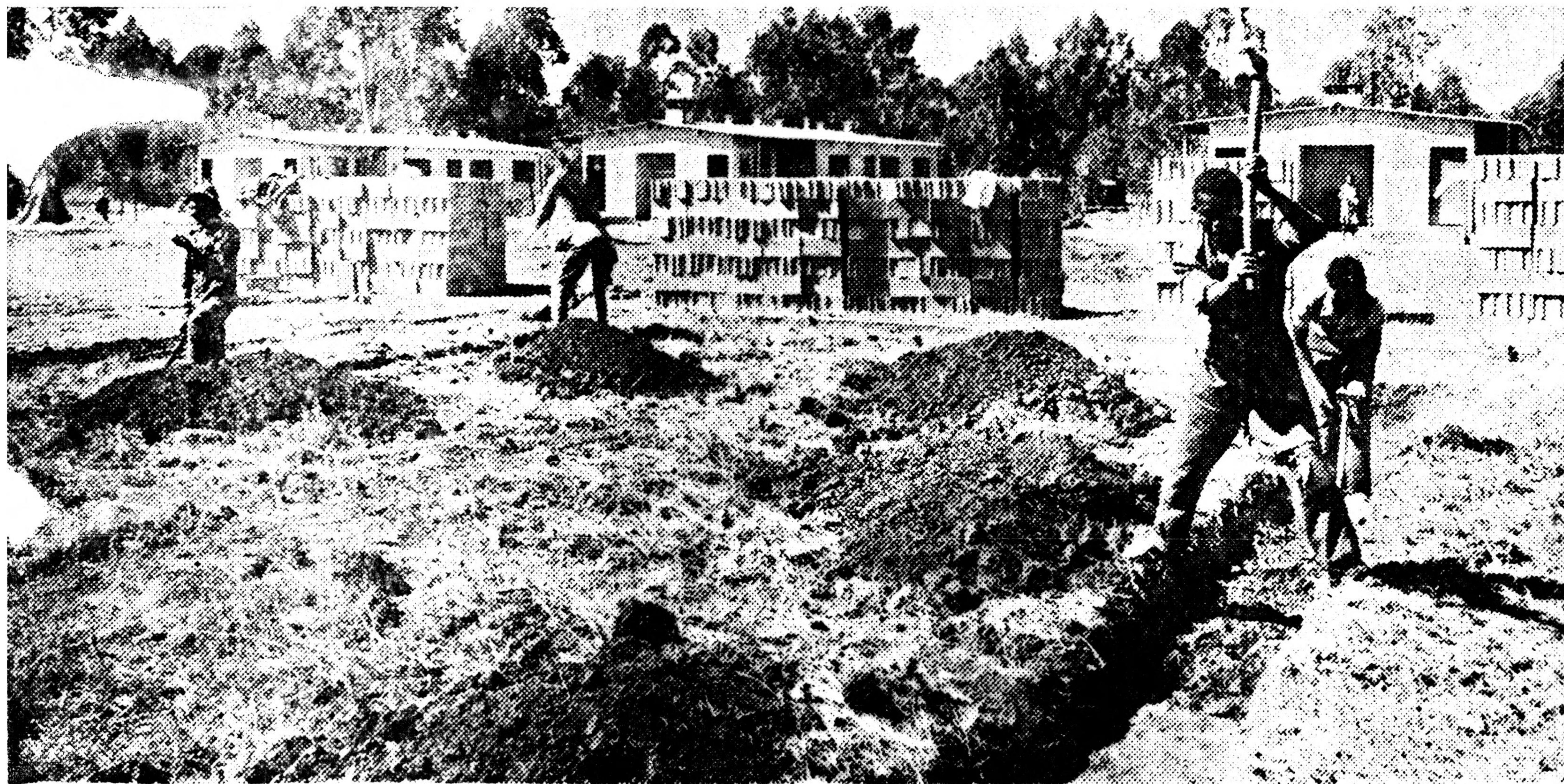
CONTRACTOR'S employees are digging the foundations for better houses for workers' families at Coolmoreen. In the background are some of the finished houses, far better than any to be found in former city townships.
