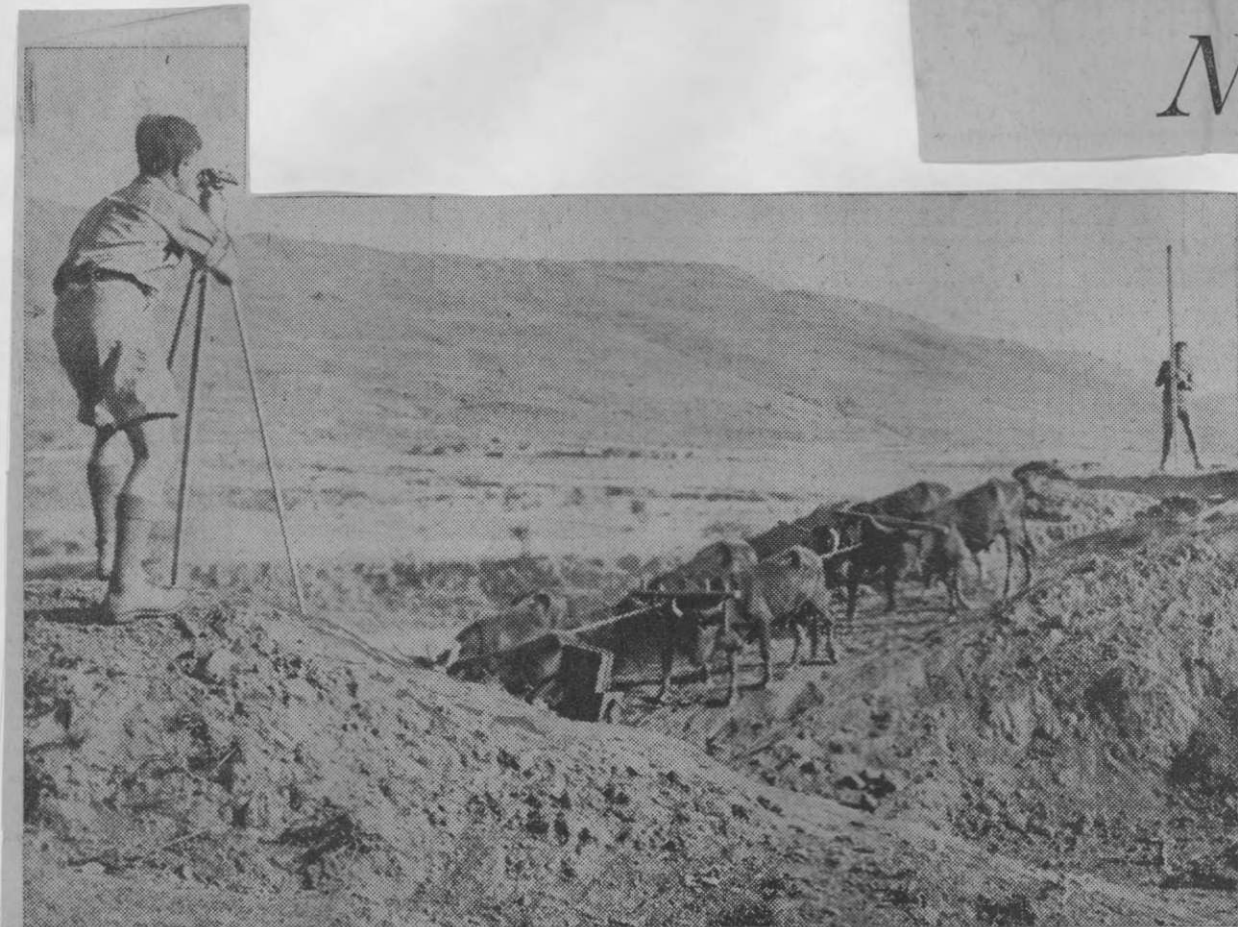
TAKING THE LEVELS on a Rietvlei farm, where 20 young South Africans are building a dam. The oxen are dragging down another load to the growing earth wall.
