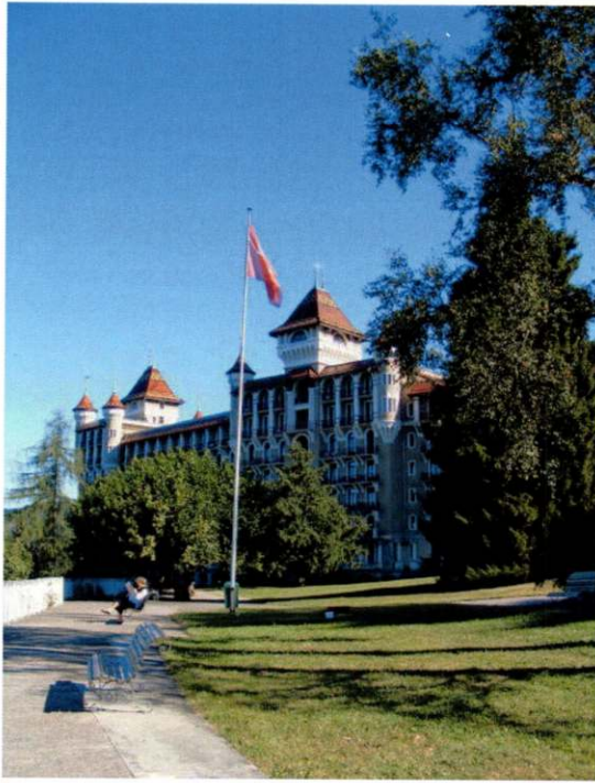
Mountain House, Caux sur Montreux, Switzerland
